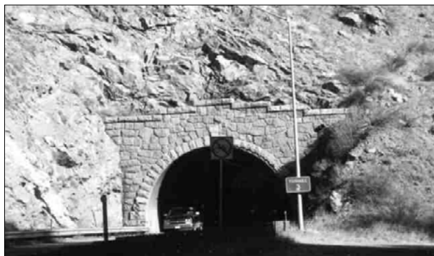
Tunnel on U.S. 6 in Clear Creek Canyon.
