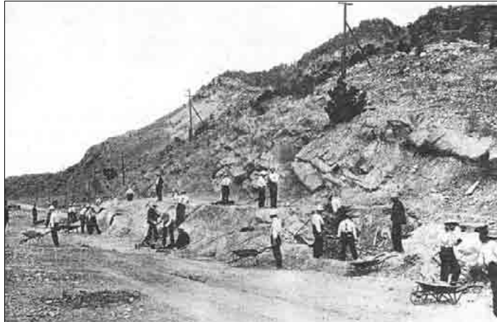
Convict road improvement project, unnamed location. Photograph from Sunlight Magazine , February 1914.
