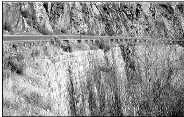
The rock benching and a stone retaining wall built by WPA workers raised the roadbed to above Bear Creek to prevent flooding.
