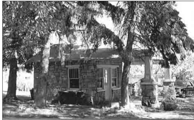
Former filling station built by John Mathews near the entrance to Mount Vernon Canyon.
